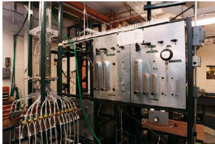
Flow distribution measurement system via collector for atmospheric pressure trickle bed reactors facility
